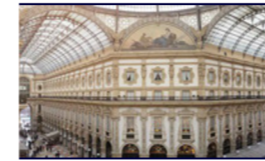
Cracco in Galleri Restaurant Milan, Italy
